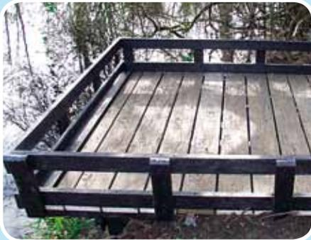
Platforms and decks constructed from recycled plastic wood composites are virtually maintenance free as they are not susceptible to damage from insects, rot or algae. Synthetic paving grids either grass seeded or packed with porous fill make a useful free draining, non-slip surface from which anglers can fish.
