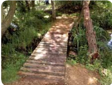
Footpath bridges are constructed to client specifications. Materials most commonly used e.g. treated soft wood, mature hard wood or synthetic timber produced from recycled plastics, are among the more popular choices.
