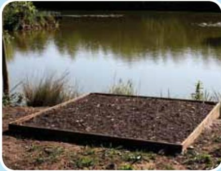
Fishing pegs will take different forms depending on the design specifications or limitations of the site. Bark chippings are an effective draining, non-slip surface. Exact positioning of the peg will often be dictated by bank characteristics and ground conditions.
