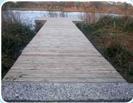
Casting platforms provide pre-determined areas where anglers can fish thus reducing both bank side erosion and potential damage caused to marginal vegetation. Platforms help to make greater areas of fisheries water accessible by effectively reducing obstructions from behind when back-casting.
