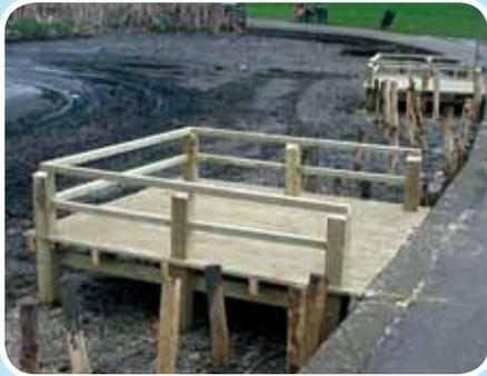
Angling platforms of treated softwood construction are built using responsibly sourced timber. Decking boards can be supplied smooth, grooved or grooved with a reeded surface. Without sacrificing the appearance of the natural wood we can, where appropriate, fit BSI recognised slip-resistant materials to reduce trip hazard.
