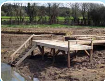
Timber bathing platforms offer a pleasing solution in providing access in and out of natural swimming ponds. The decking creates space for kit, seating and viewing. A.G.A. structures are each constructed to suit practical, fiscal and aesthetic criteria.
