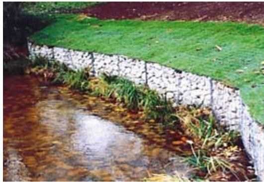
Gabions form a flexible monolithic structure and can maintain total structural effectiveness even on land liable to differential settlement.
