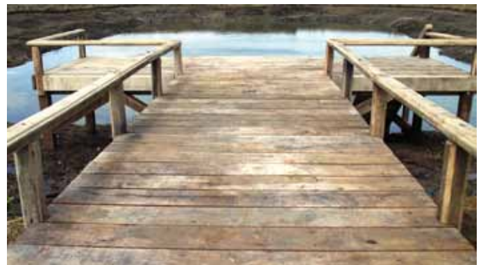
Following our design for the staging, A.G.A. craftsmen built the platform structure on site with oak plank flooring and oak balustrades. Treated softwood was used for the underwater supports giving sufficient platform height to allow natural water movement thus keeping a viable habitat beneath.
