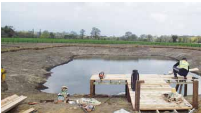
Following our design for the staging, A.G.A. craftsmen built the platform structure on site with oak plank flooring and oak balustrades. Treated softwood was used for the underwater supports giving sufficient platform height to allow natural water movement thus keeping a viable habitat beneath.
